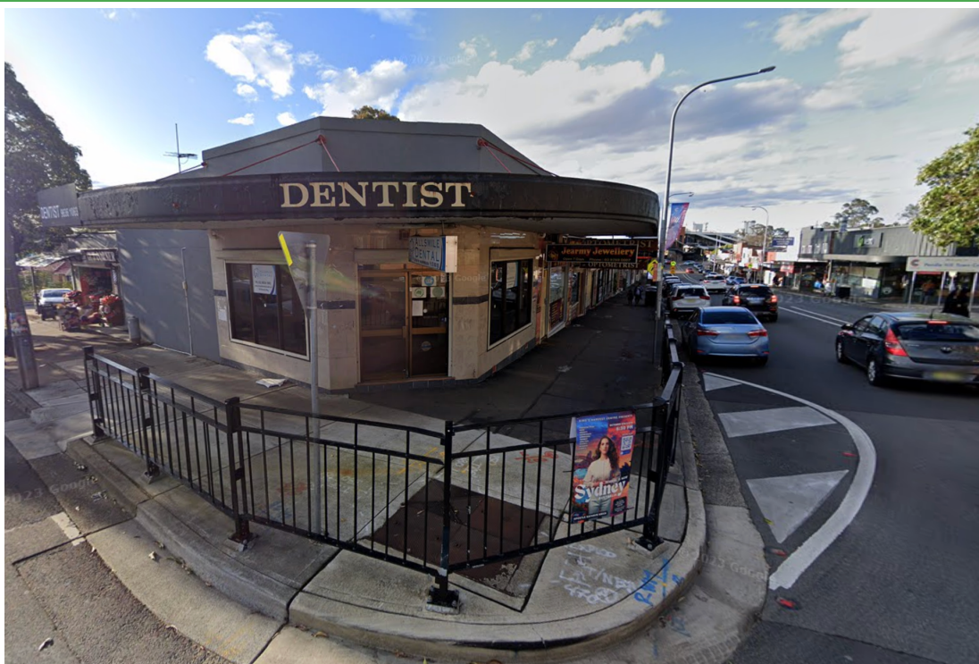
Photograph 4: shows the existing commercial precinct on the corner of Gilba Road and Pendle Way
